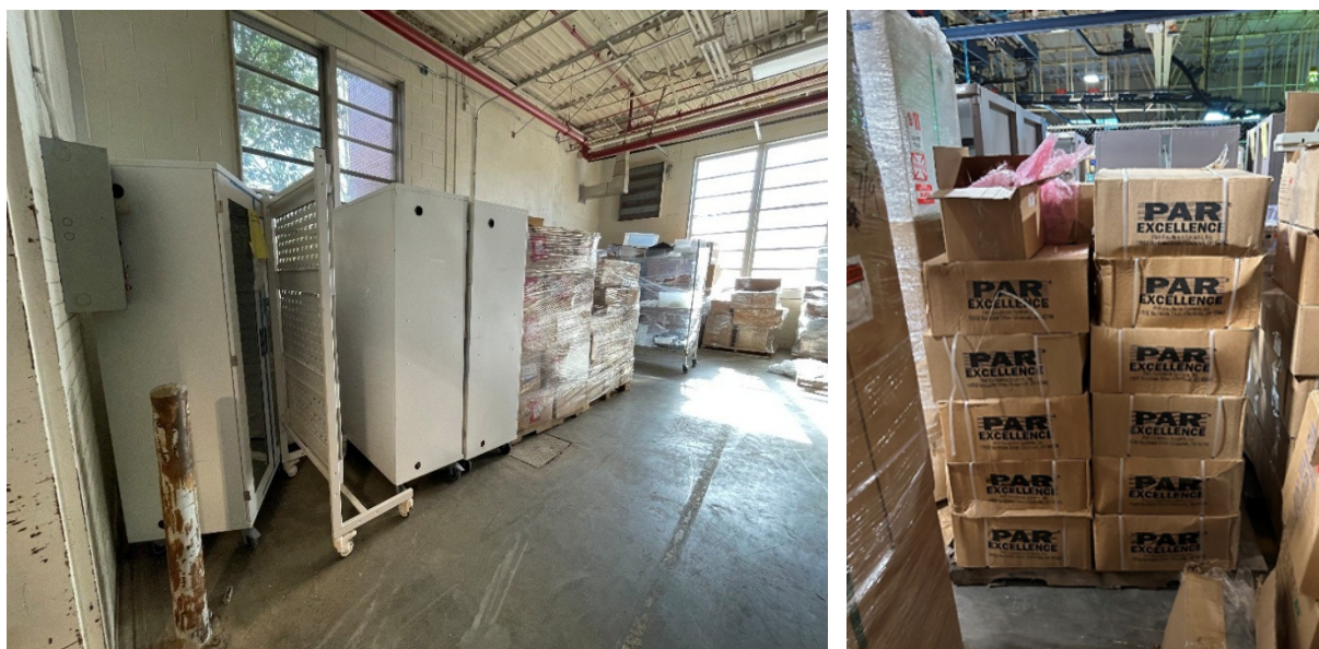
Figure 3. PAR Excellence cabinets (left) and boxes of PAR Excellence equipment (right) stored in a warehouse at the VA Augusta Health Care System.
