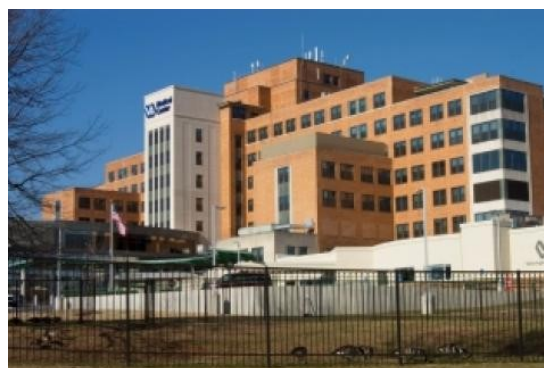
Figure 1. Facility photo. Source: “Wilmington VA Medical Center,” VA, accessed February 3, 2026, https://www.va.gov/wilmington-health-care/locations .
