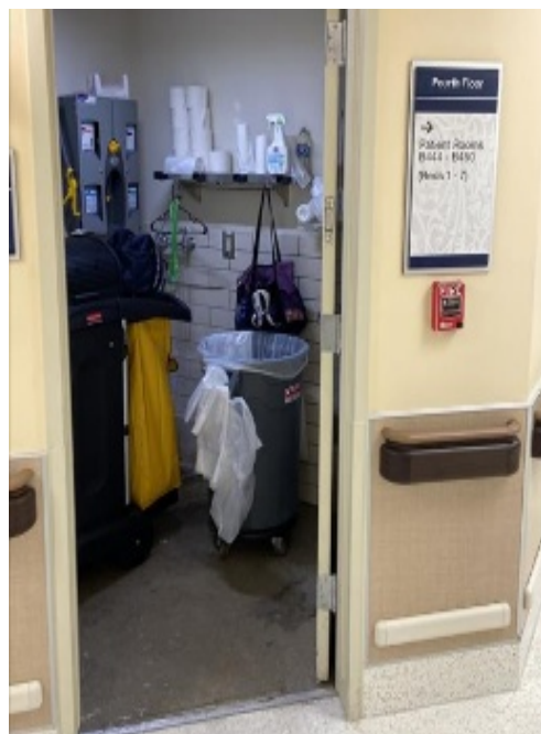
Figure B.3. Unattended environmental services cart that propped open a door to a custodial closet containing cleaning supplies and equipment.
