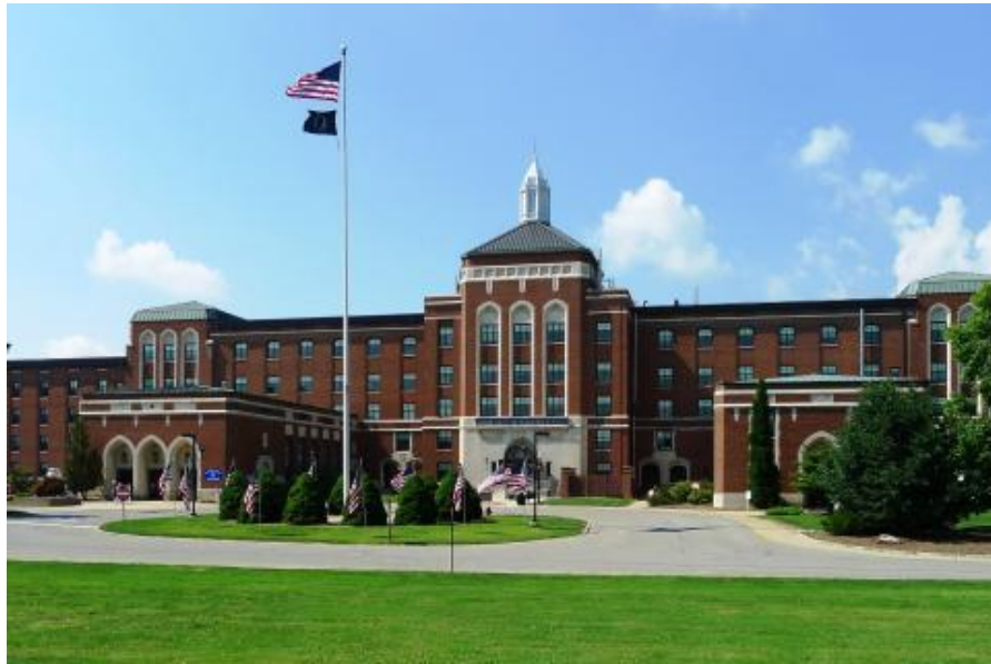
Figure 1. Butler VA Medical Center of the Butler VA Health Care System in Pennsylvania.
