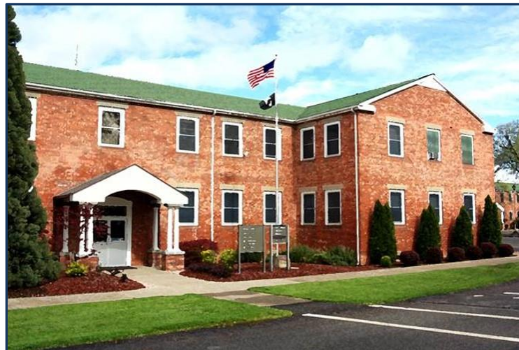
Figure 2. Southern Oregon Rehabilitation Center and Clinics.
