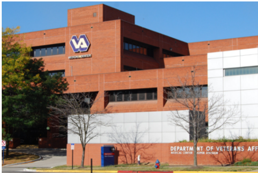
Figure 1. Lexington VA Health Care System in Kentucky.
