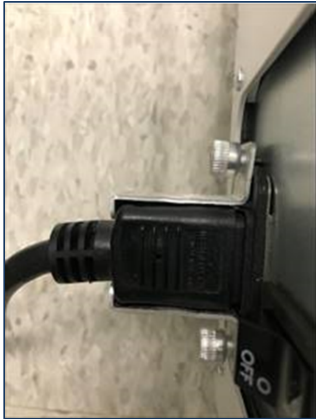
Figure 1. Refrigerator or freezer plug secured with a plug lock at the Jamaica Plain VA Medical Center.
