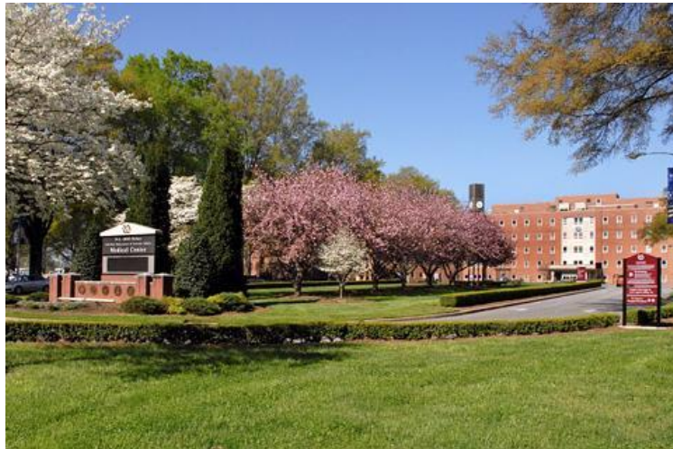
Figure 1. W.G. (Bill) Hefner VA Medical Center in Salisbury, North Carolina.
