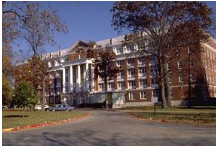
Figure 1. VA Illiana Health Care System in Danville, Illinois (Source: https://vaww.va.gov/directory/guide/ , accessed on January 28, 2020)
