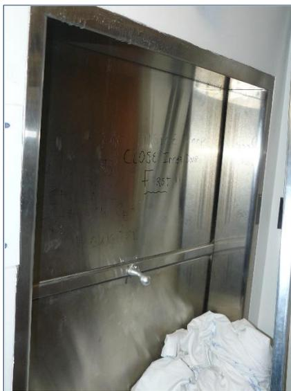
**Figure 13.** A photo of an unlocked dumbwaiter in a telecommunications room.
