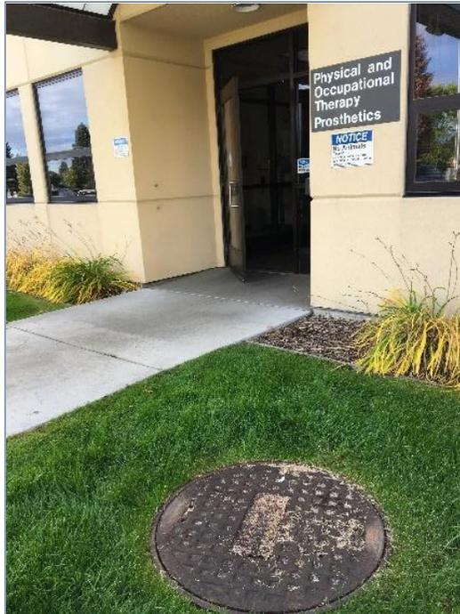
**Figure 11.** A photo of the unsecured maintenance manhole located on the Mann-Grandstaff VAMC campus taken by the team during the OIG site visit. All fiber cabling for the campus runs through this maintenance manhole.
