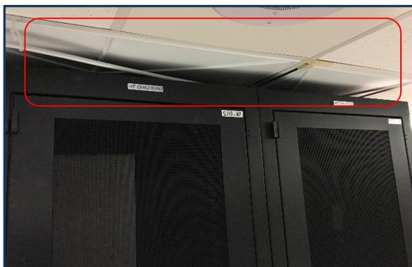
**Figure 9.** (Right) Picture shows the ceiling tiles installed directly above server racks, which will eventually hold Cerner's servers. The tiles are used to prevent equipment damage that could be caused by leaking pipes above.
