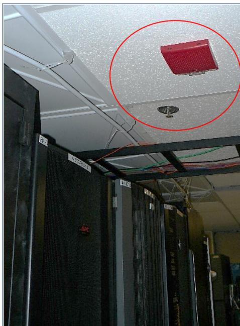
**Figure 8.** (Left) Picture of the proximity of the sprinkler heads to the server racks in the data center room, taken during the audit team's inspection.
