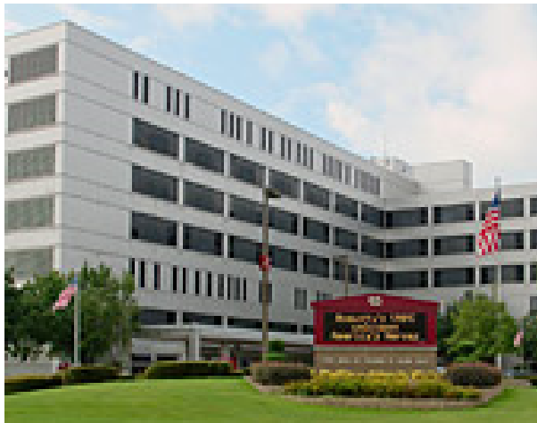
Figure 1. Charlie Norwood VA Medical Center, Augusta, Georgia (Source: https://www.augusta.va.gov , accessed on July 23, 2019)
