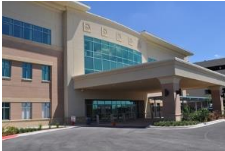
Figure 1. VA Texas Valley Coastal Bend Health Care System, Harlingen, Texas (Source: https://vawww.va.gov/directory/guide/ , accessed on May 30, 2019)
