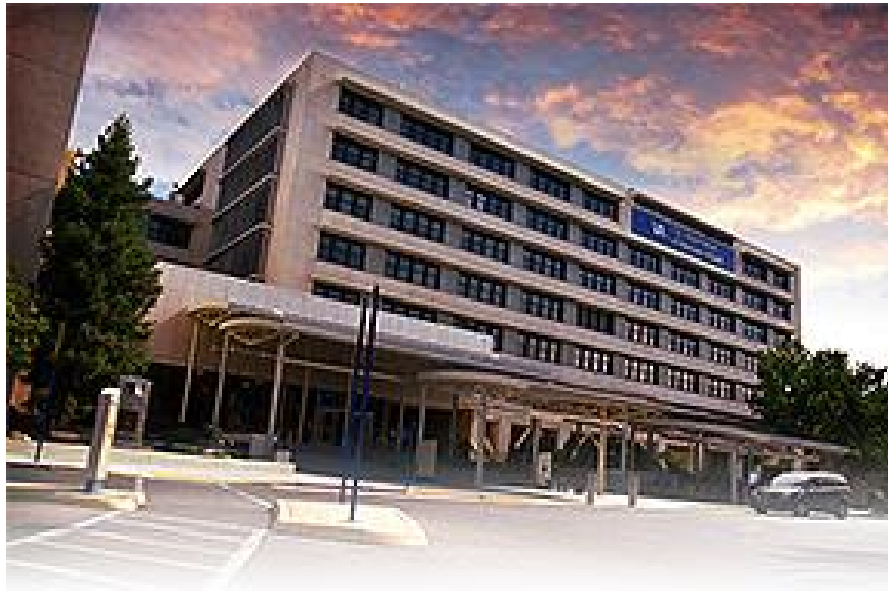
Figure 1. Central California VA Health Care System, Fresno, CA (Source: https://vaww.va.gov/directory/guide/ , accessed on April 23, 2019)
