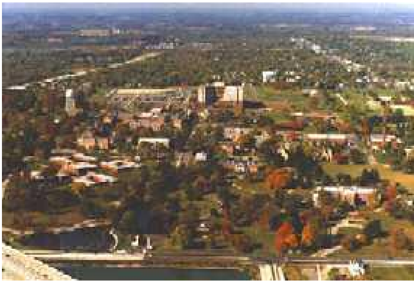
Figure 1. Dayton VA Medical Center, Dayton, Ohio (Source: https://vaww.va.gov/directory/guide/ , accessed on May 23, 2018)
