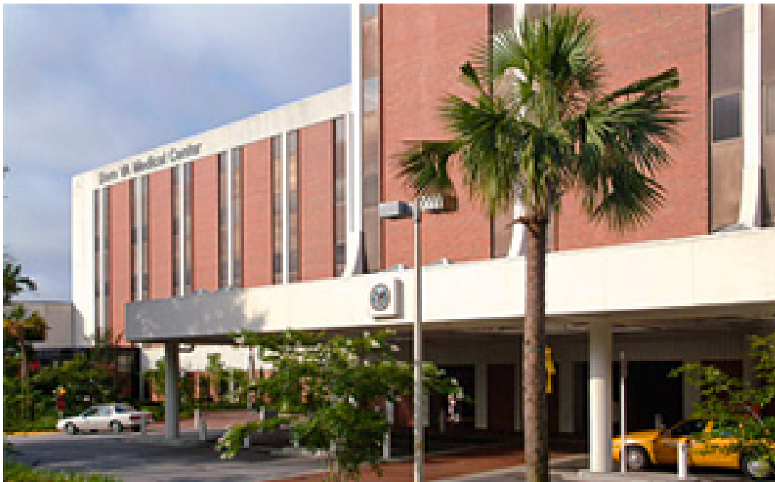
Figure 1. William Jennings Bryan Dorn VA Medical Center, Columbia, South Carolina (Source: https://vaww.va.gov/directory/ . Accessed on April 19, 2018.)
