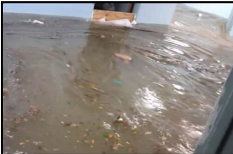
Figure. Ground Floor Flooding and Damage
