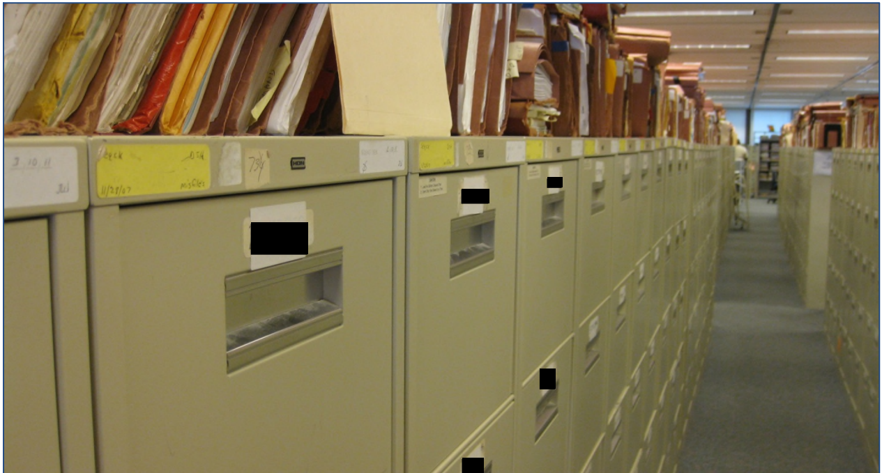
Figure 3 – File cabinets show gradual sloping away from support structures
