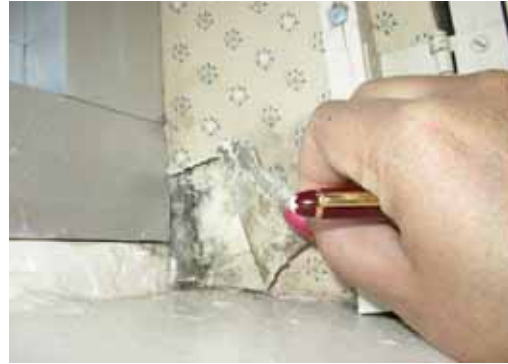
Photograph 1. Mold behind wallpaper in the dining room.
