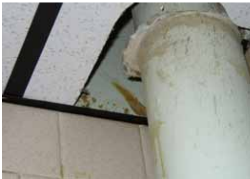
Photograph 2. Unsealed opening in ceiling of food storage area.
