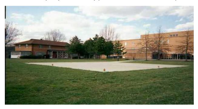
The helicopter pad has not been evaluated for safety issues such as obstacle clearance (buildings, trees, etc.), weight bearing capacity (capability to support helicopter dropping onto pad), and foreign object damage resulting from concrete chipping or other matter.
