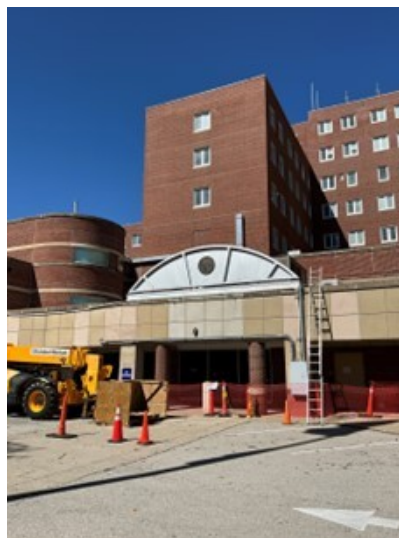
Figure C.4. Unattended ladder at clinic entrance.
