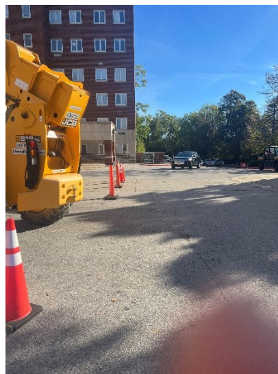
Figure C.2. Photo of drive-up ramp to clinic entrance.
