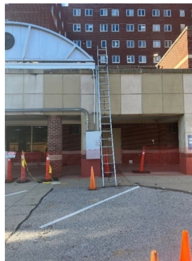
Figure C.5. Unattended ladder at clinic entrance.
